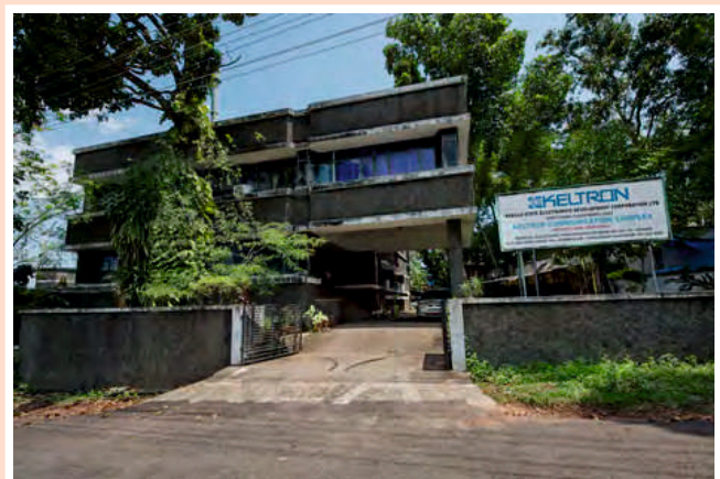
Keltron Communication Complex (KCC) Monvila, Trivandrum
