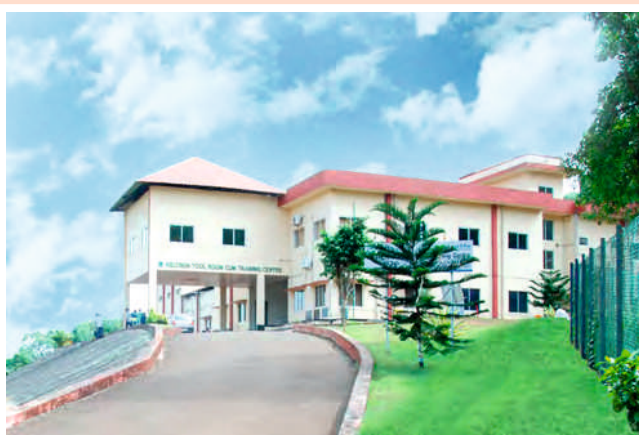
Keltron Tool Room cum Training Centre, Kuttippuram Malappuram
