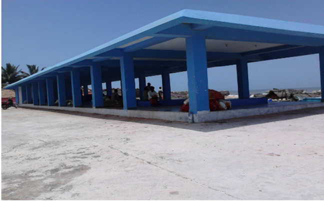
Fish Landing Centre, Paruthiyoor, Trivandrum
