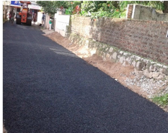
Kalleluvayal Road, Kollam
