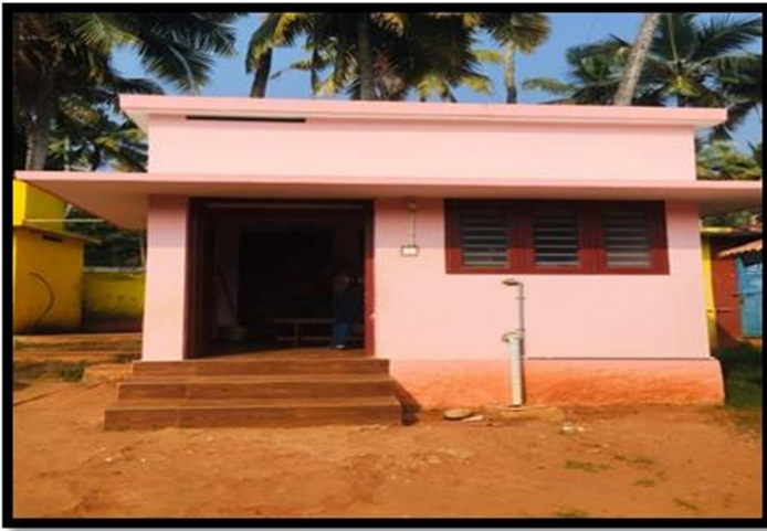
GLPS, Pulluvila GLPS, Kitchen shed, Trivandrum
