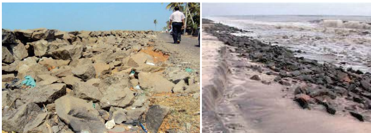
Eroded Sea wall
