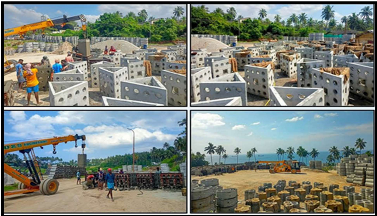
Image 2. Casting of Reefs in progress
